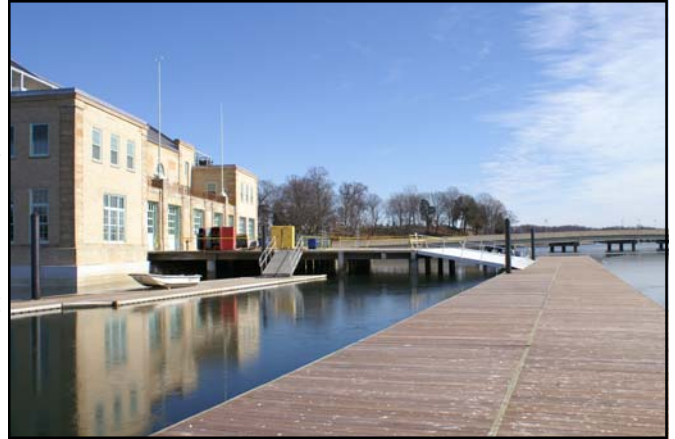
Newly installed dock and ramp for Hubbard Hall
