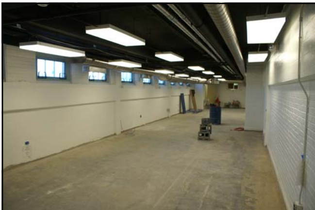
New 3rd Deck Erg Room/Visiting Team Locker Room
