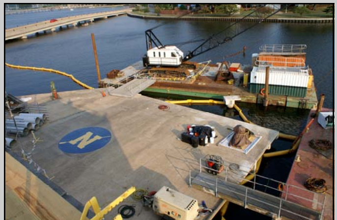
Dock and Apron Under Construction
